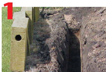
1 Dig a channel (5" deep and at least 8" wide). Set sod carefully aside for reinstallation.
