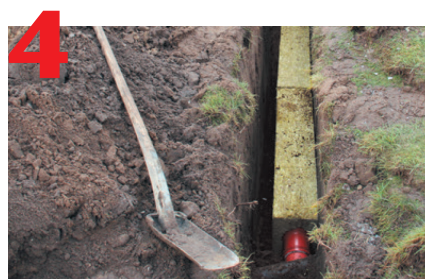
4 Backfill the trench with removed soil.
