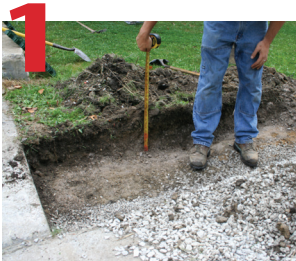
Excavate area. Set curb, or other edging, if required.
