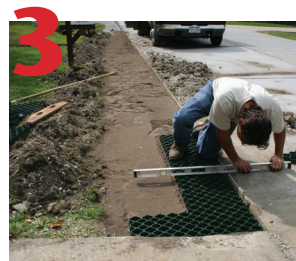
Spread sand over the bedding layer, compact well. Position GrassGrid and ensure everything is level.
