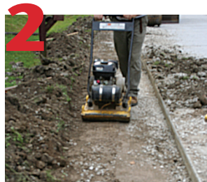
Spread fill/bedding layer evenly, compact well.
