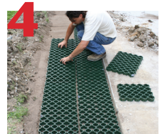
Continue to lay GrassGrid. Click parts together and stagger joints. Use anchor nails on perimeter grids (2 per grid). For extra security (especially on slopes) use additional nails on interior grids where desired.
