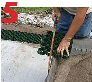
GrassGrid is easily cut using a hacksaw.
