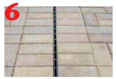
Lay remaining channels, units slide-fit together. Finish pavement/pavers must be an 1/8" higher than edges of drain. Bond pavers to cover and concrete haunch to prevent damage to slot when trafficked.
