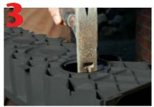
Knockout channel base for outlet at required position.
