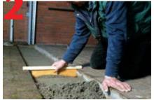
Lay 4" deep concrete bed. Cut channels to fit required length (if necessary).
