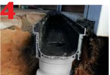
Push-fit outlet adaptor into bottom of channel, lav outlet channel first and connect to 3" or 4" SDR pipe or 4" schedule 40. Alternatively, use 4" flex coupling to connect 4" SDR pipe to outlet on base of corner unit, set in place and lay channels from that point.
