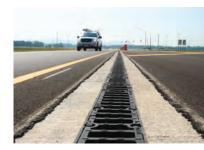
Trench drainage provides continuous capture and simple one-way grades to ensure an effective solution with easier installation.
